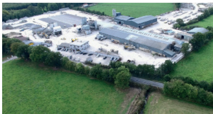
Figure: Ducon Concrete Ltd.
